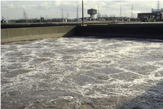
(a) Beckton STP, Activated Sludge Tank. John Ros-tron, CC BY-SA 2.0
